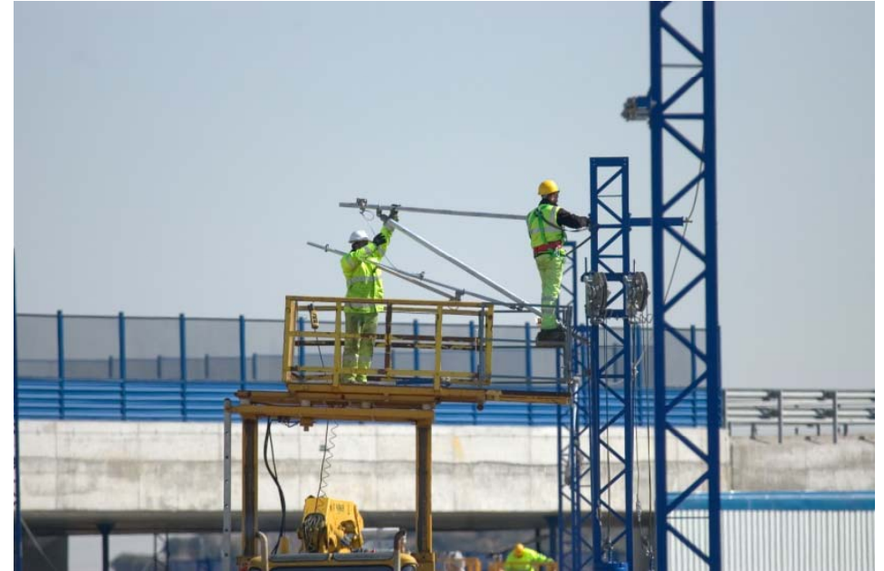
Installation without crane (approx. 35 kg/cantilever), only 2 workers on platform needed
